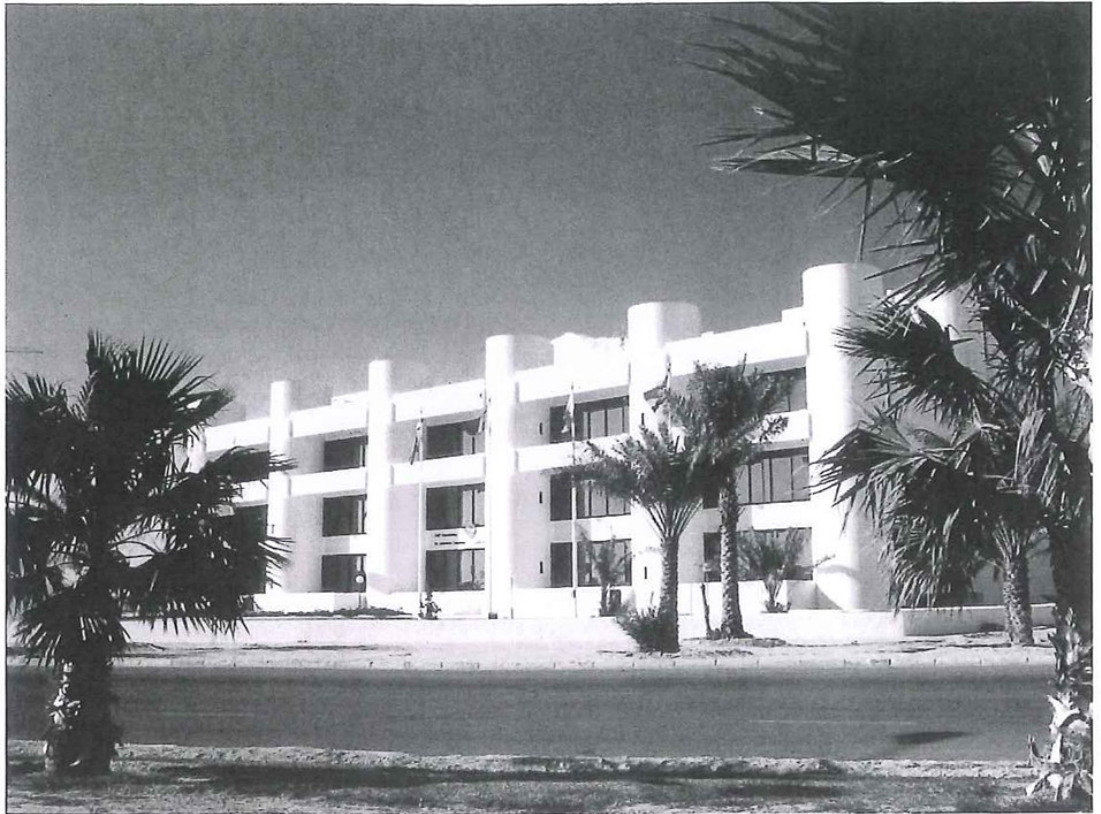
John S. Bonnington Gulf Organization for Industrial Consulting (GOIC) headquarters Doha, Qatar 1984 Courtesy: John S. Bonnington, London
